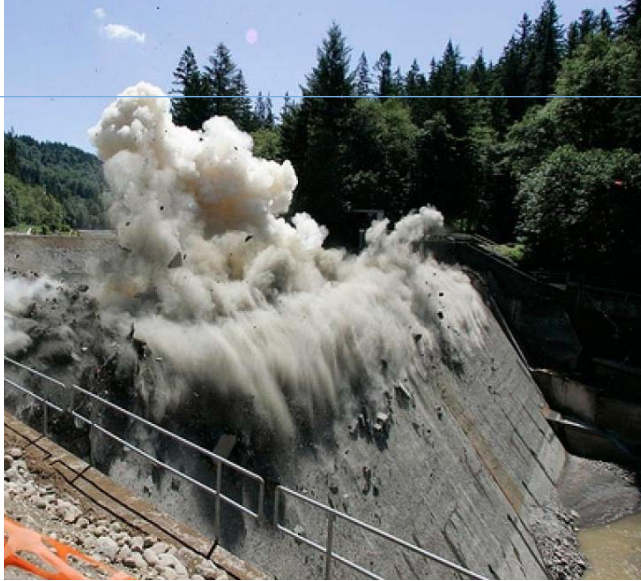
2007 removal of the Marmot Dam, Sandy River, Oregon. Photo: NOAA
